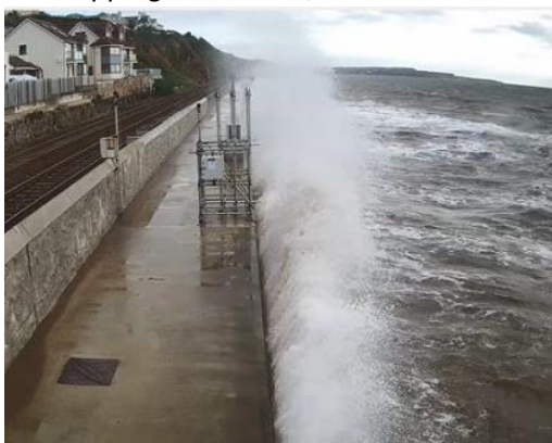
Overtopping at Dawlish, 7 th March 2022
