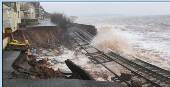
Damaged railway lines at Dawlish, 2014
