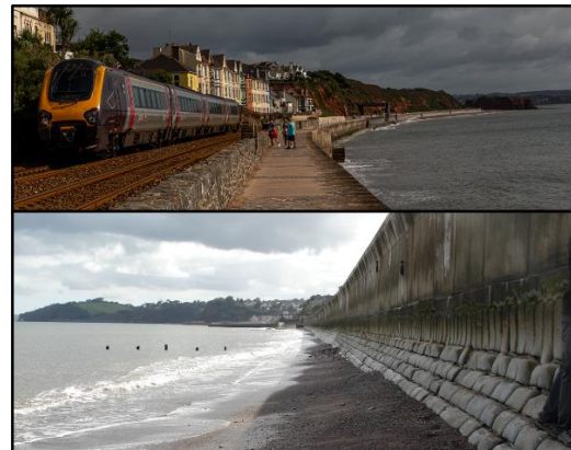
The Dawlish train line, walkway and sea wall
