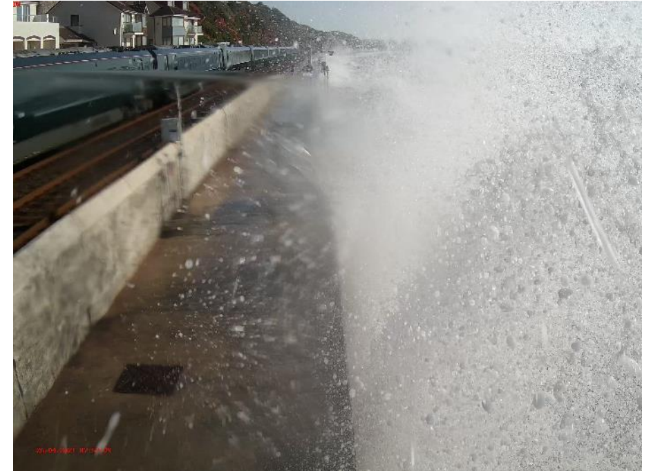
Wave overtopping hazard, being measured by the CreamT project in Dawlish, April 2021. University of Plymouth camera footage.
