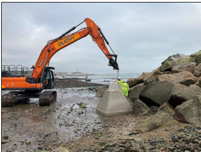
88 eco-blocks have been installed around the rock armour breakwater
