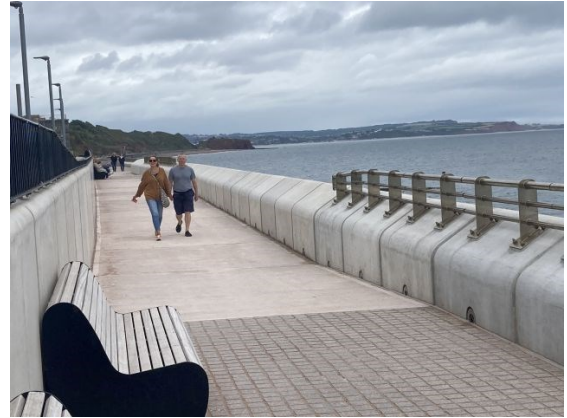
New promenade and sea wall at Dawlish — photo: Paul Berry
