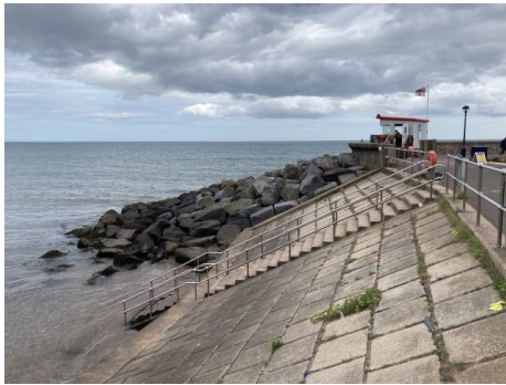
Revetment & rock armour — photo: Paul Berry
