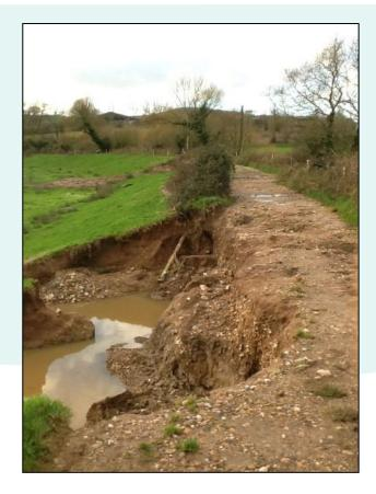
In March 2018, flooding caused severe erosion of embankments built to protect agricultural land from flooding.
