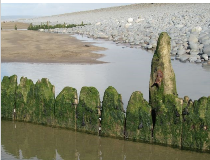
Old groynes —photo: Paul Berry
