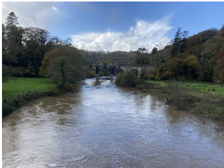
Canal Bridge Aqueduct —Photo: Paul Berry
