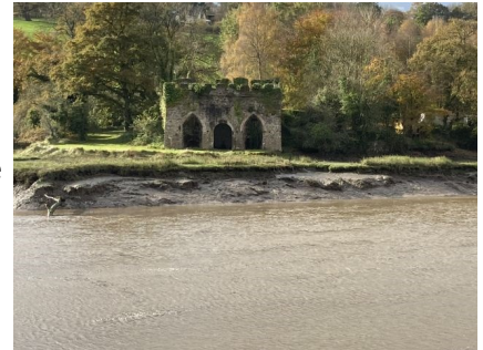
Lime kilns at Iron Bridge —Photo: Paul Berry
