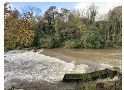
Weir at Beam Bridge —Photo: Paul Berry
