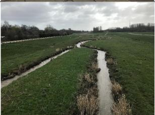
Re-wilding of the 1970s Marsh Barton flood relief channel, with new year-round meandering river created. During normal flow, most river water follows the main River Exe channel which is behind the trees on the left of this picture. When a flood occurs, water pours over a spillway and fills up the flood relief channel, which doubles the capacity.
