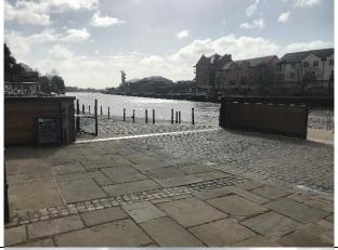
New flood gates at the downstream end of the Quay protected area, outside the Waterfront Pizza restaurant. Upstream from here, removable steel flood barriers can be slotted into pillars when high river flows are likely. Businesses downstream will rely on flood proofing techniques and individual building protection.
